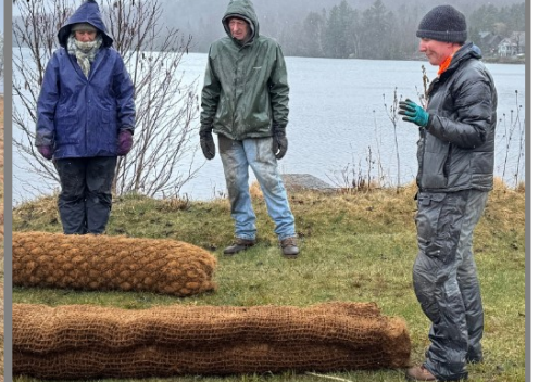
BioD-Blocks and Coir Logs used to prevent Shore Erosion
