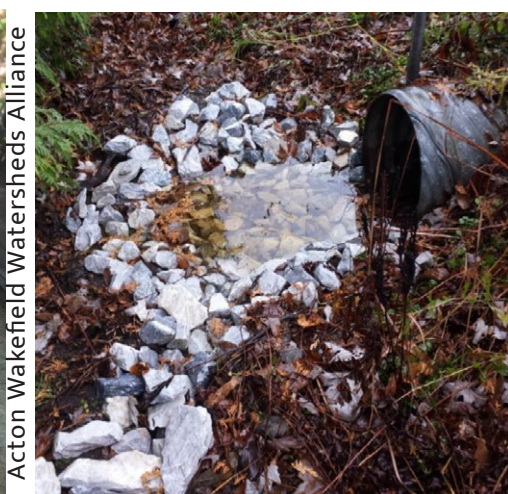
Small rock apron at culvert outlet.
