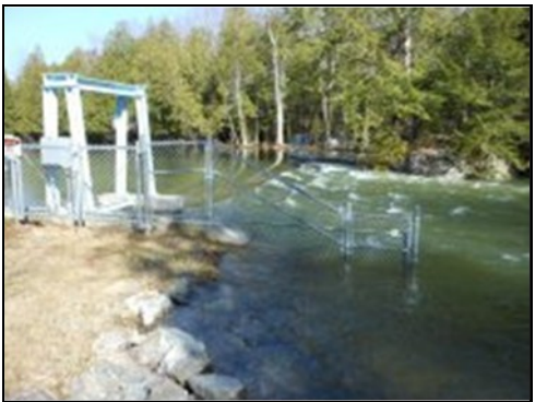
The present dam during extremely high water level. The tall iron structure on the left contains a moveable gate at the bottom.
